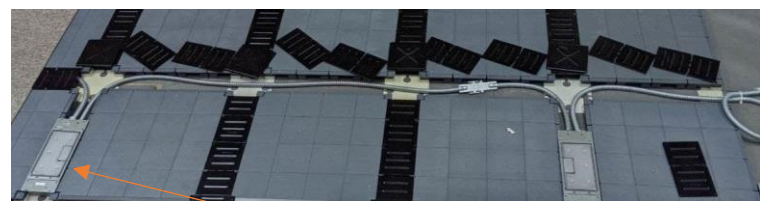
series connection and extension of floor boxes.
